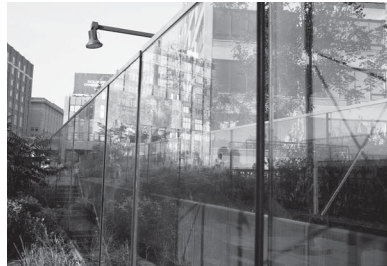
PAGES 134–45: James Corner Field Operations and Diller Scofidio + Renfro, The High Line, section 1, 2009
